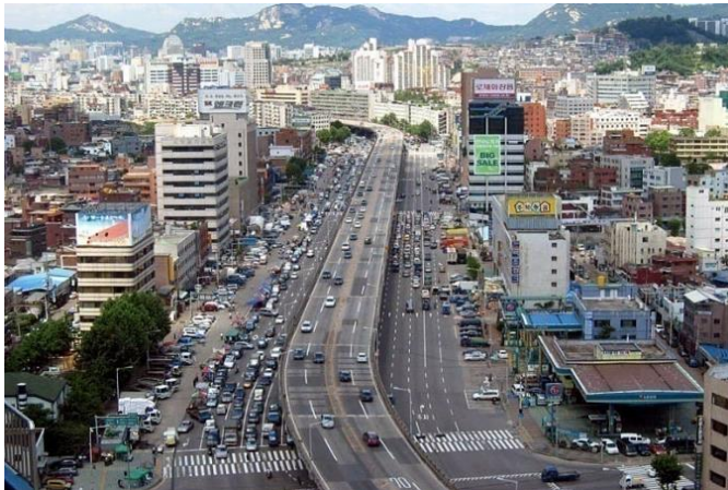
June 2003 Before Restoration
