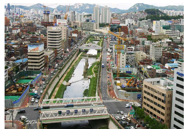
September 2005 After Restoration
